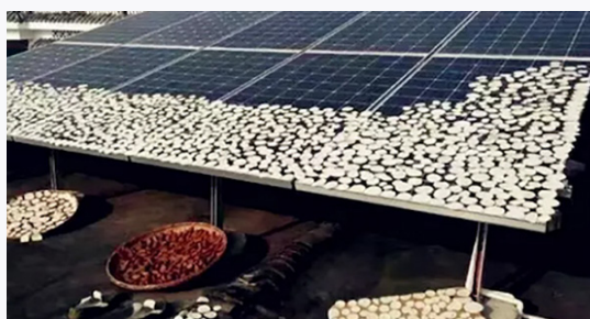
Figure 50: Shading due to drying crops
