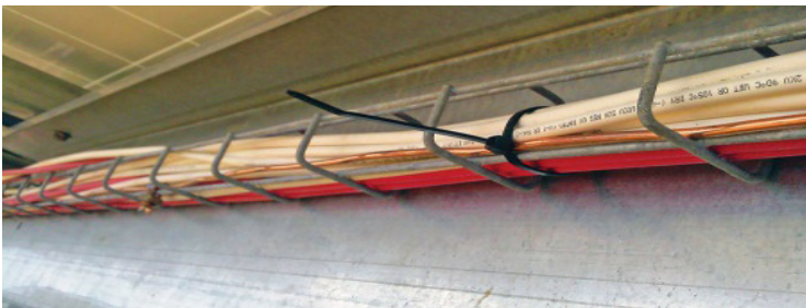
Figure 113: Cables are tied using cable tie
