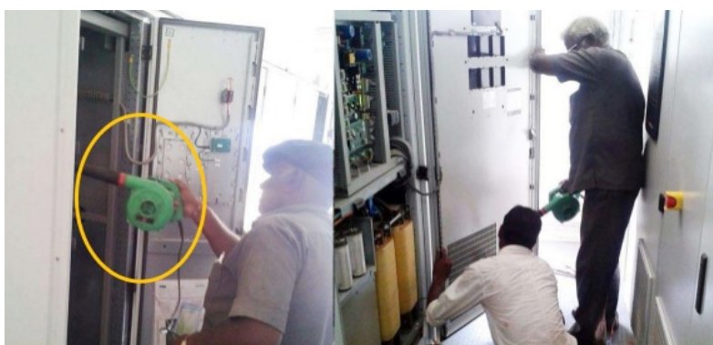
Figure 89: Cleaning inverter using blower
