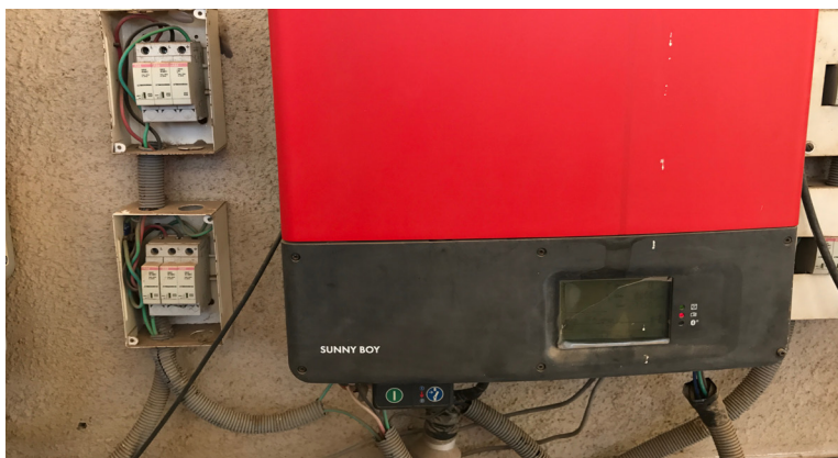
Figure 86: Inverter cables and conduits got loosed
