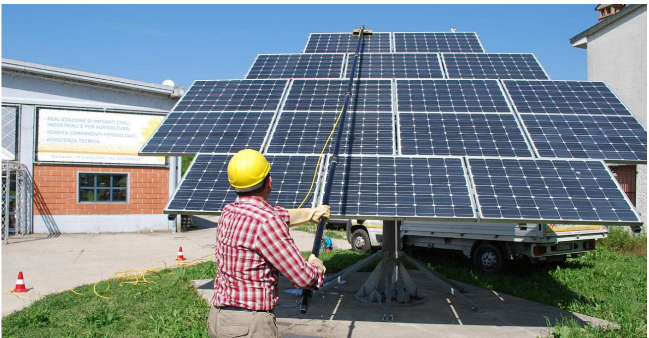
Figure 37: Wet Cleaning (Manual)
