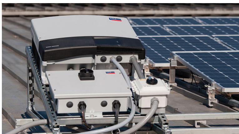
Figure 84: Inverter installed without any shade or roof
