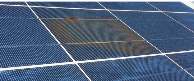
Figure 35: Corrosion
