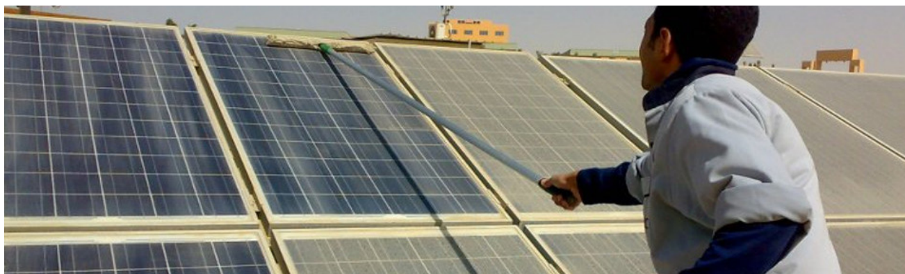
Figure 42: Dry Cleaning Method (Manual)
