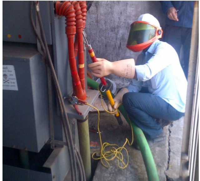
Figure 155: Correct practice - With face shield
