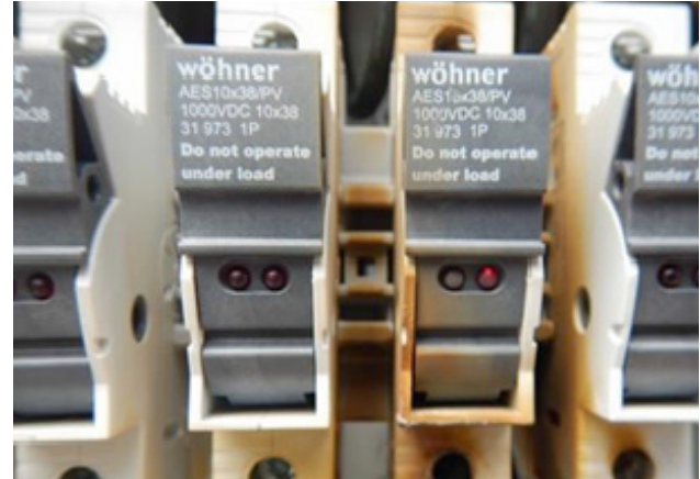
Figure 120: Fuses - Burnt out
