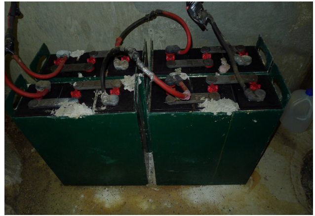
Figure 127: Improper condition of battery
