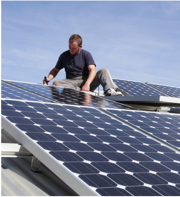
Figure 160: Incorrect practice - Without safety belts
