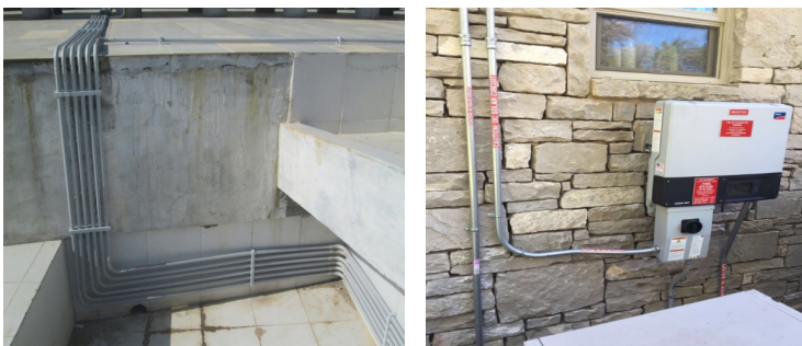
Figure 101: Proper cable routing
