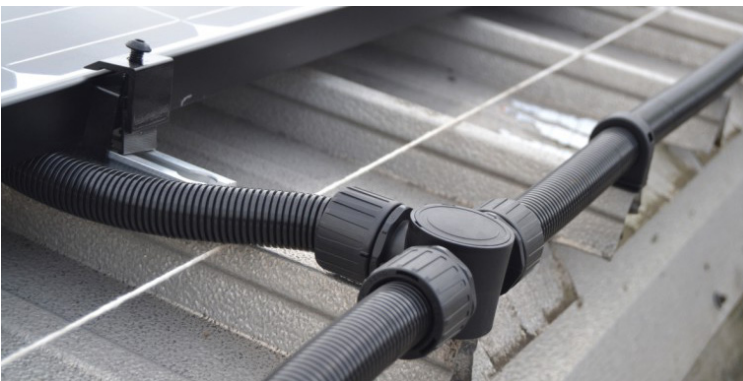
Figure 110: Correct - Conduits are in proper condition
