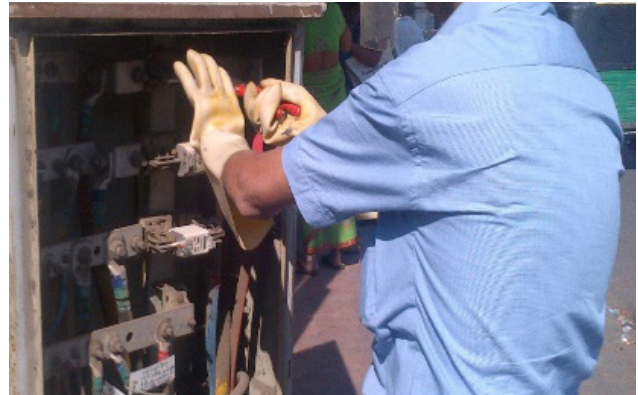
Figure 159: Correct practice - With safety gloves
