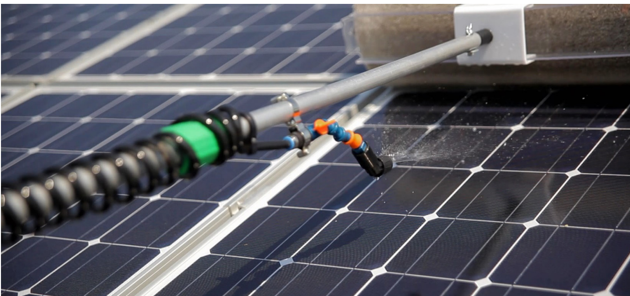
Figure 45: Wet cleaning using an automated system
