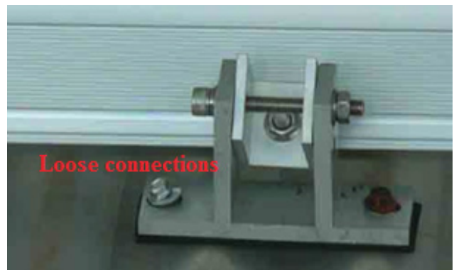
Figure 118: Loosed clamps
