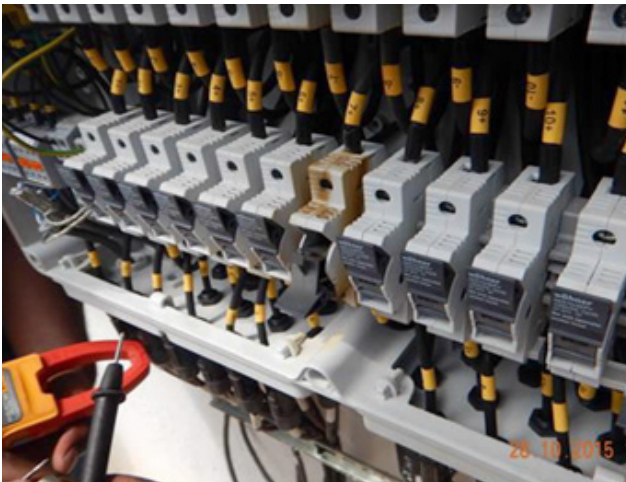
Figure 140: Testing using clamp meter
