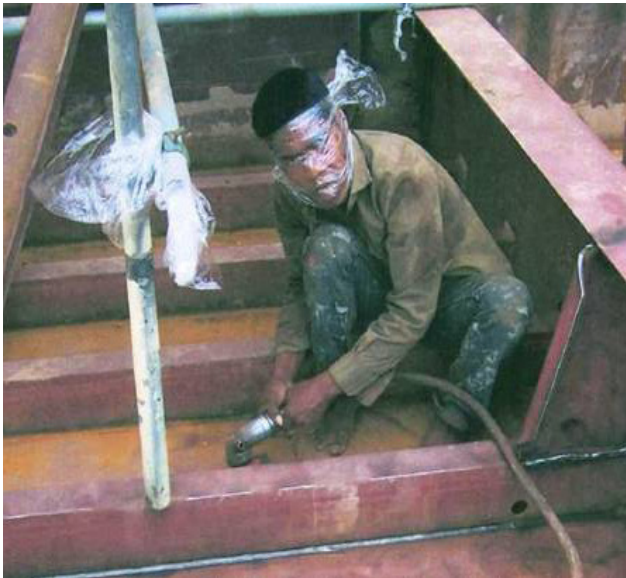
Figure 154: Incorrect practice - Without face shield
