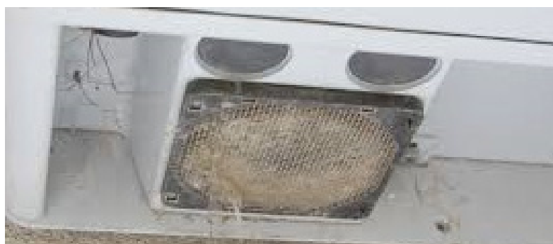
Figure 88: Dust accumulation on Inverter
