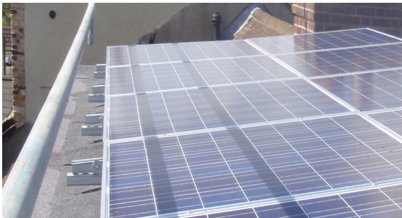
Figure 51: Shading due to nearby poles on terrace
