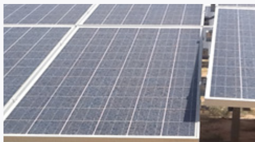
Figure 48: Nearby module casts a shadow on another module
