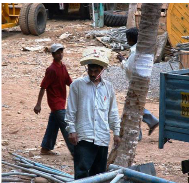
Figure 150: Incorrect practice - Without safety helmet
