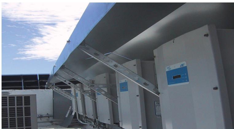
Figure 85: Inverter installed under shade
