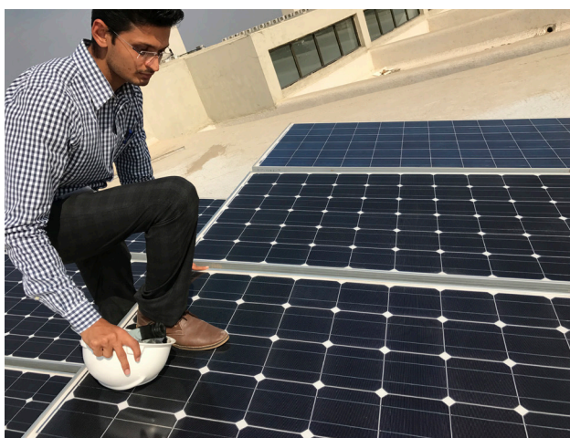
Figure 40: Never sit or stand on PV modules
