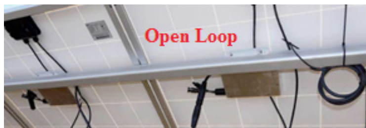
Figure 103: Incorrect cables connection looped loosely
