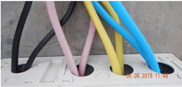
Figure 107: Incorrect – Cable conduit are not closed
