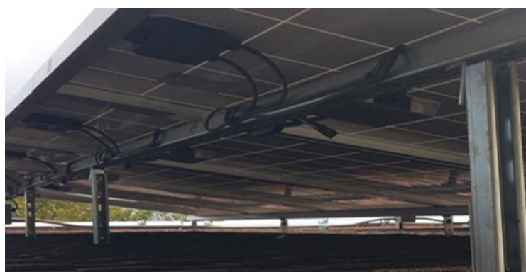
Figure 104: Correct cabling connection
