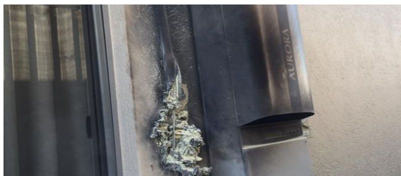
Figure 81: Inverter damage - Burn out
