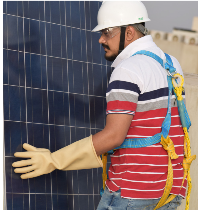
Figure 161: Correct practice - With safety belts
