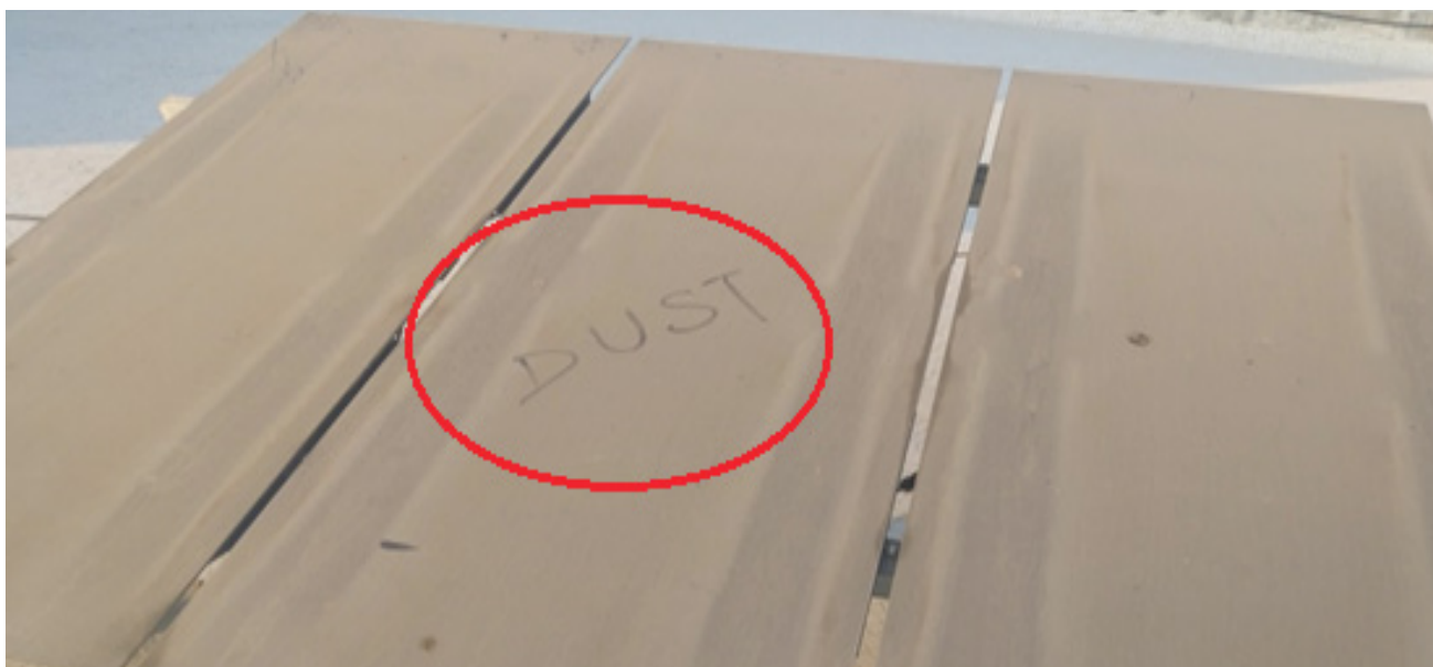
Figure 25: Cleaning required (Significant financial impact)
