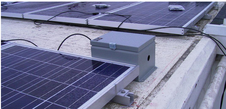
Figure 100: Incorrect cable routing
