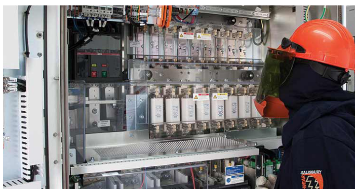
Figure 92: Check inverter fuses
